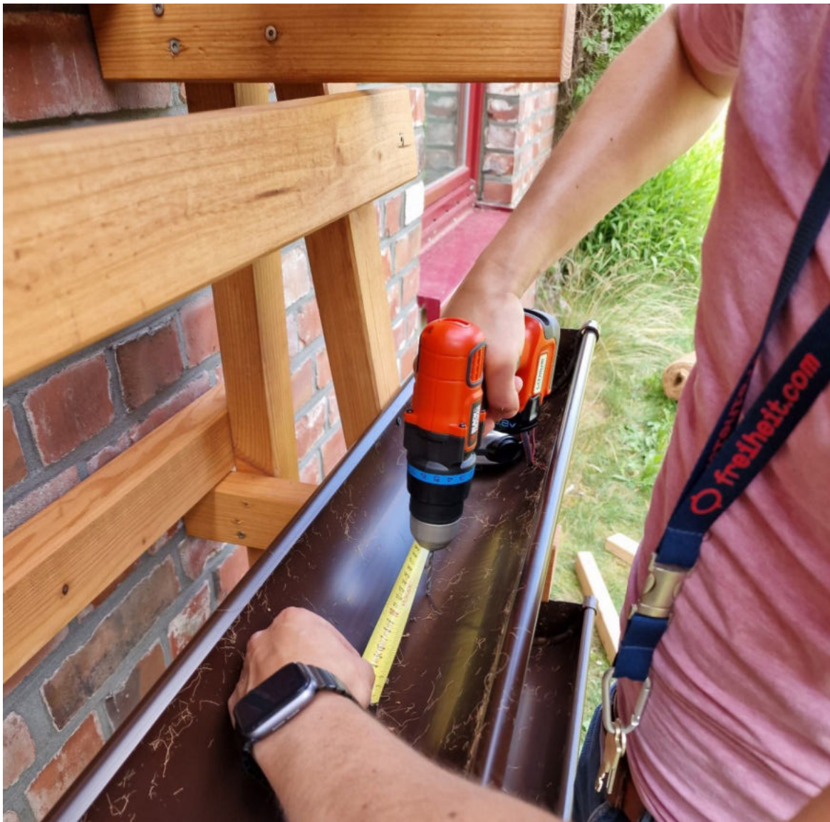
Figure 24: Drilling the drainage holes.
