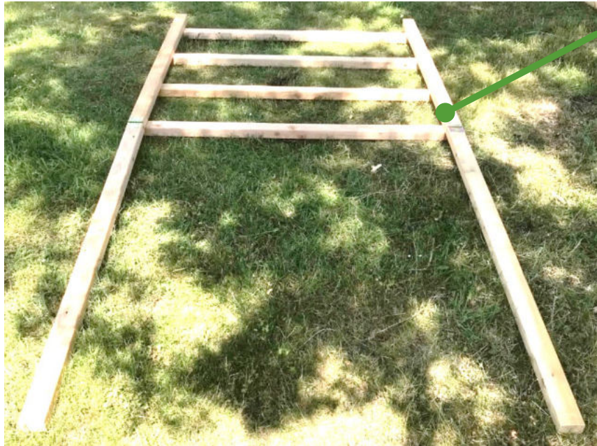
Figure 13: Assembling of the front frame.
