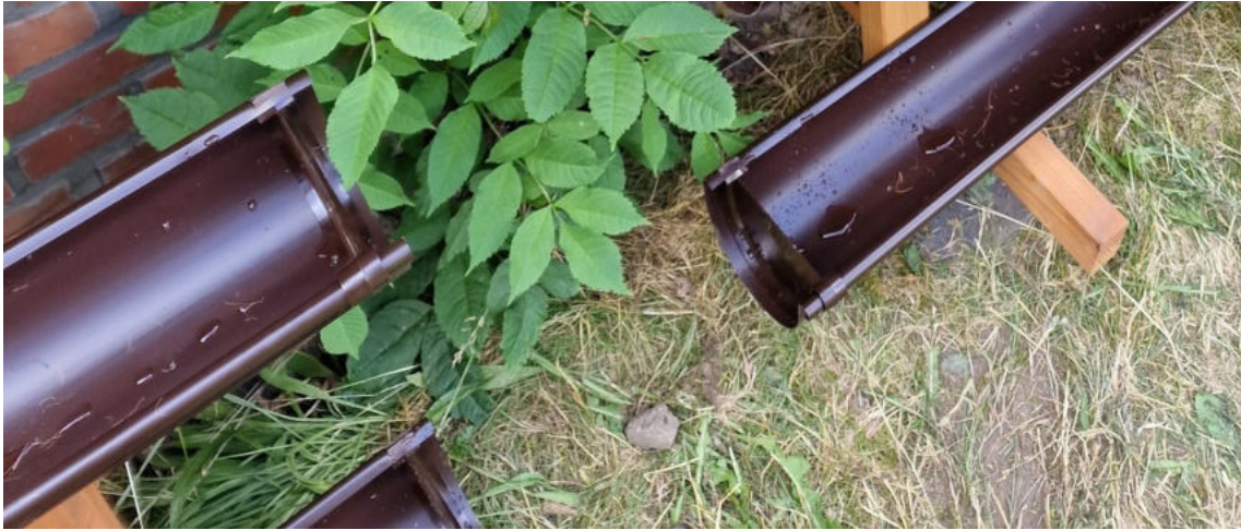
Figure 22: Rain gutters fastened to the frame.
